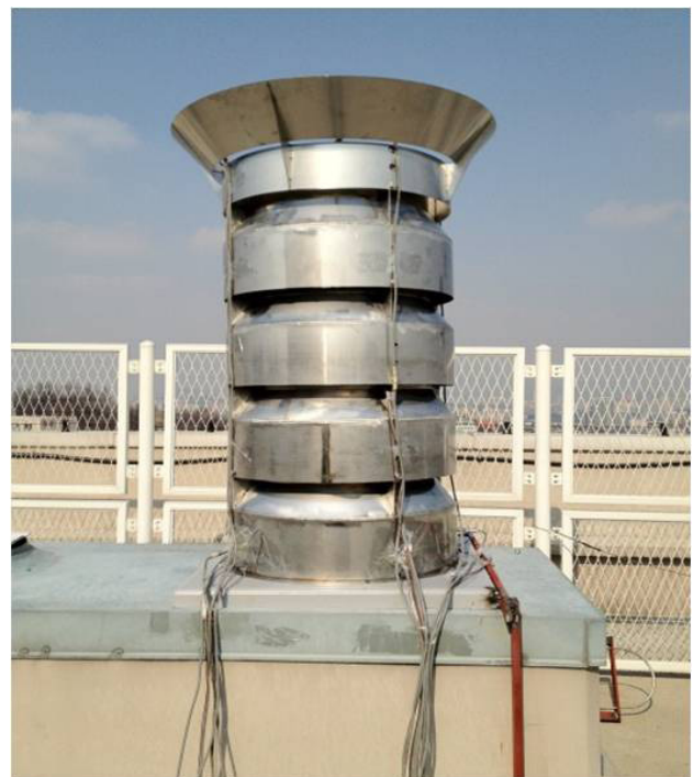
Fig.10. Installation of Mock-Up Model on Exhaust
