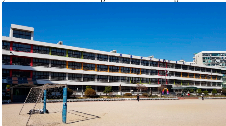
(b) School building in 2019
