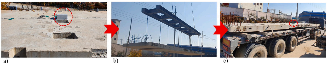
Fig. 5. a) PDMS positioned on the PCS in the GR stage, b) AL stage monitoring, and c) TR stage.
