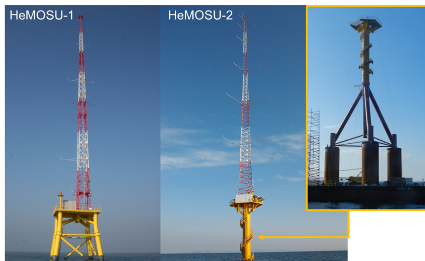
Fig. 5. Offshore meteorological masts with different types of substructures in the yellow sea of Korean Peninsula.
