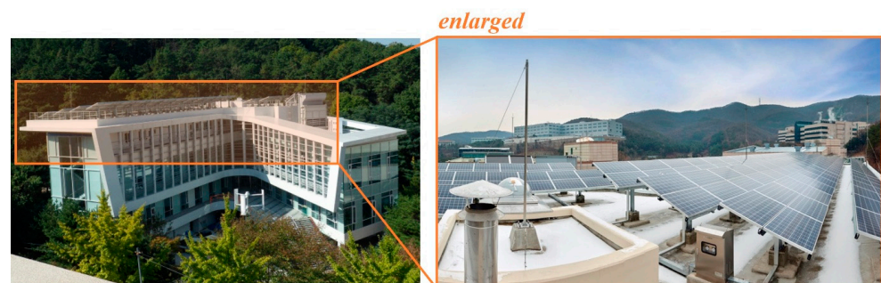
Figure 2. General view of building-integrated photovoltaic (BIPV) generation system.
