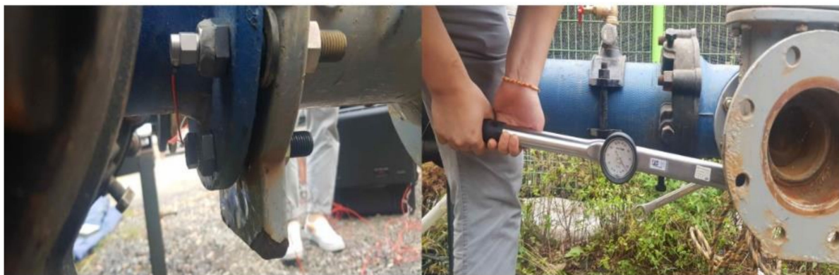
Figure 6. Smart bolt installation and measurement of torque.
