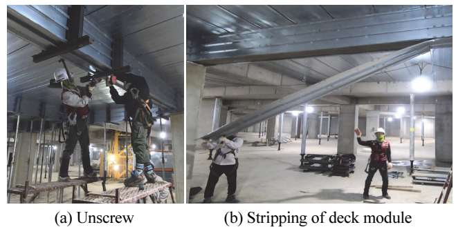
Fig. 12 Removing process of beam-deck form
