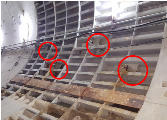
(a) Check-valve for grouting confirmation
