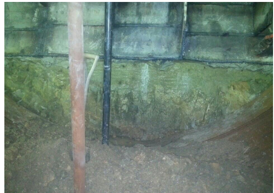
(b) Removal of steel segment bottom before thrust
