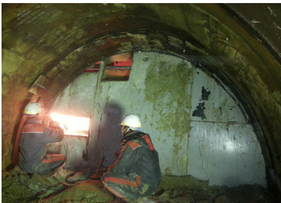
(c) Removal of steel segment after thrust
