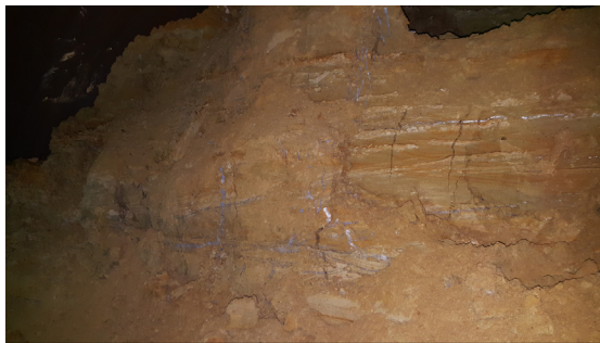
(a) Cross-connection tunnel 2 (04/13/16)
