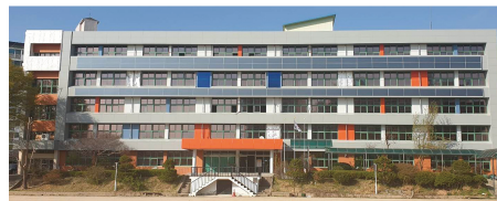
After facade renovation with BIPV
