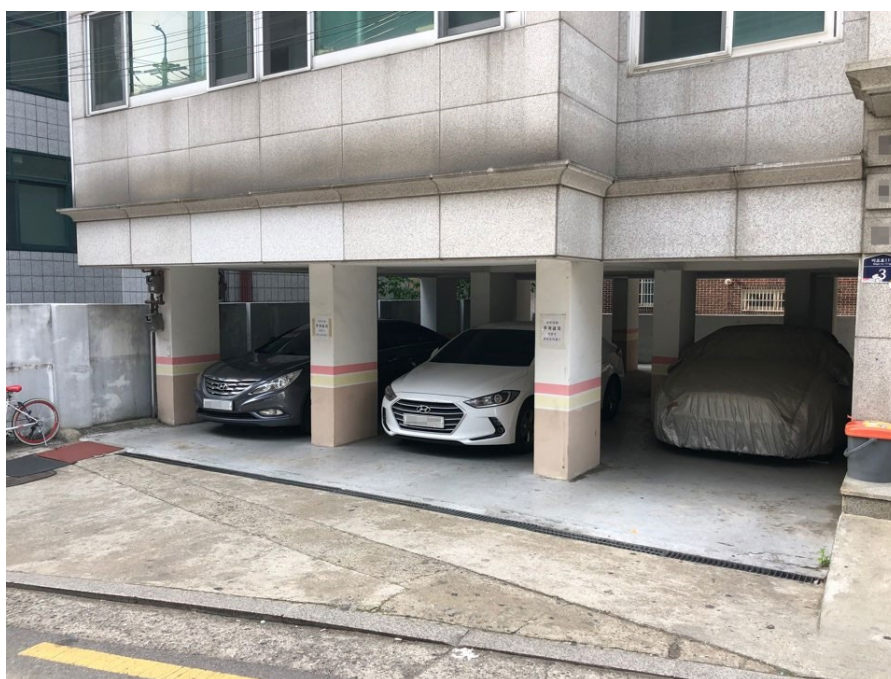
Figure 1. Piloti structures used to make parking space in Korea.
