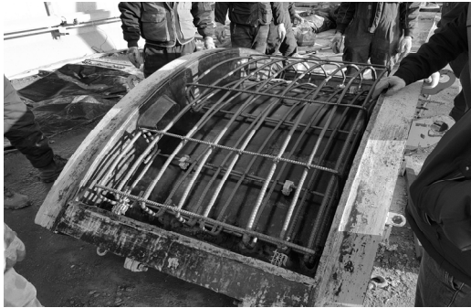
(a) Steel bar in a segment mould
