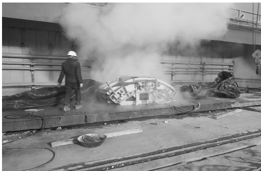
(c) Steam curing
