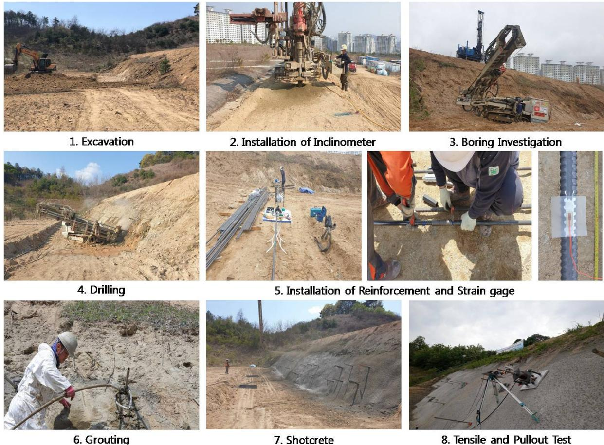
Fig. 6. Flow of a field test construction
