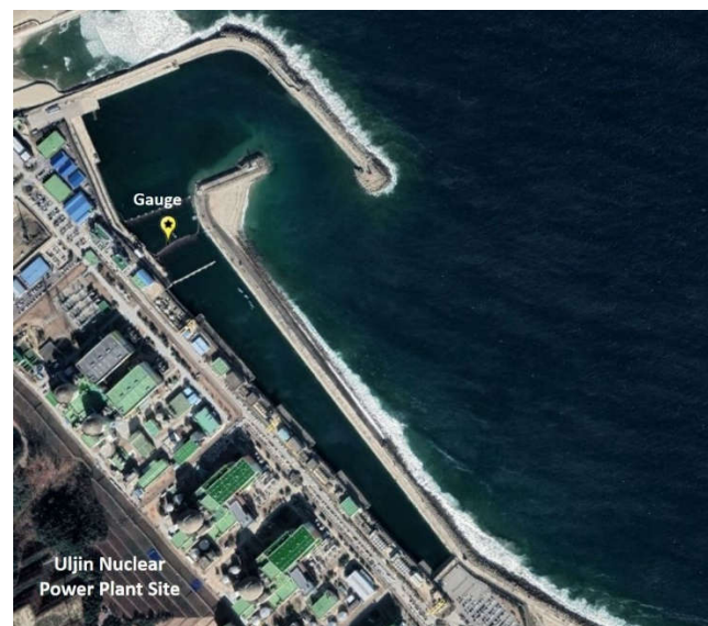
Figure 6. Location of gauge in Uljin Nuclear Power Plant.
