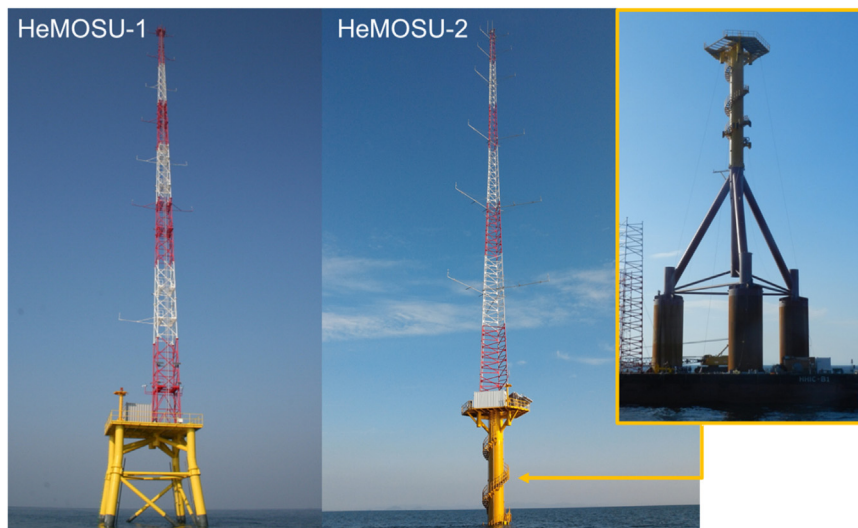
Fig. 5. Offshore meteorological masts with different types of substructures in the yellow sea of Korean Peninsula.
