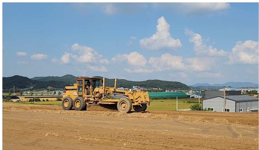
Figure 15. Motor grader working along the generated path.
