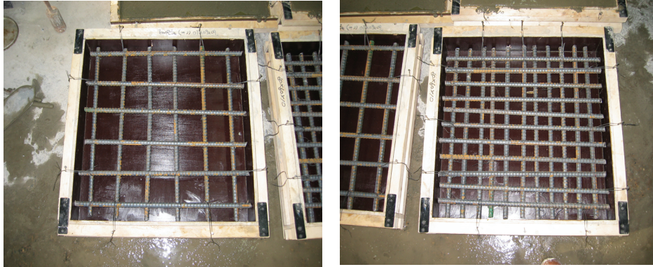
FIGURE 4: Placement of bars (D16@10, D16@5).
