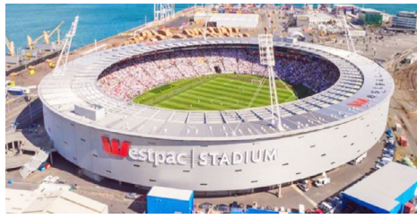
d) Wellington Westpac Trust Stadium, New Zealand
