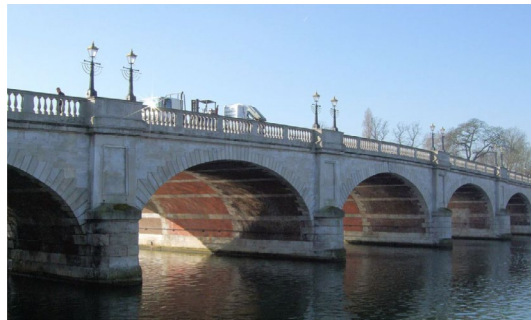
b) Kingston Bridge, England
